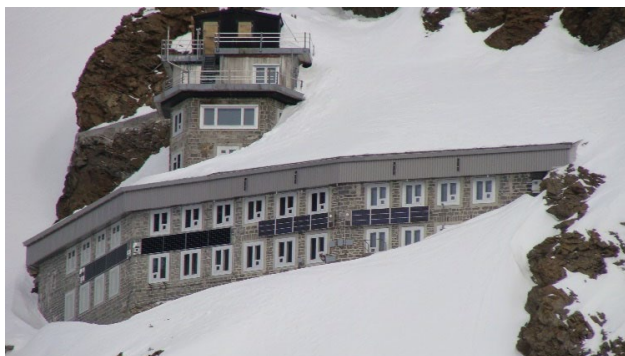
Figure 1. PV system at Jungfrauoch
