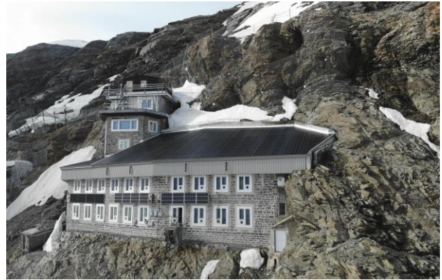
Figure 4. PV system at Jungfrauoch in Summer 2023
